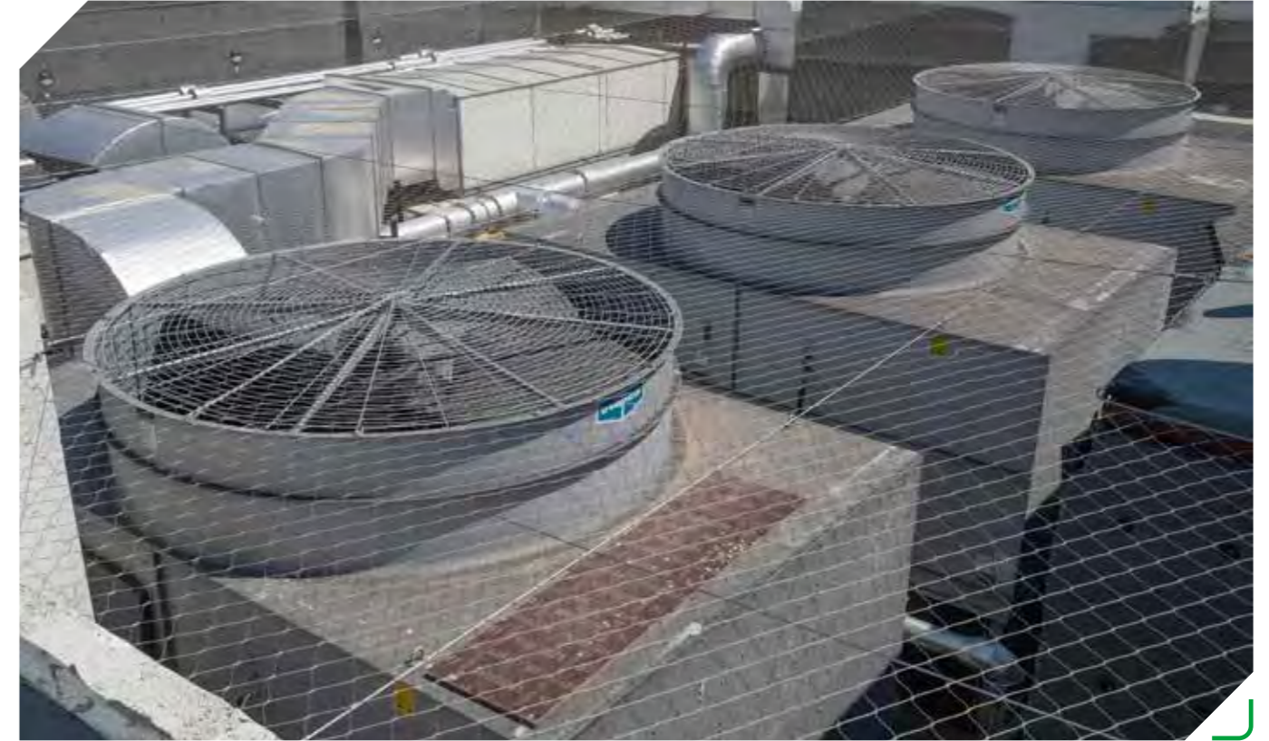
► Gallery Lines, boiler room and TSB buildings, all engineering and mechanical field works of Samsun City Hospital with a construction area of 300,000 m 2 and a capacity of 900 beds.
