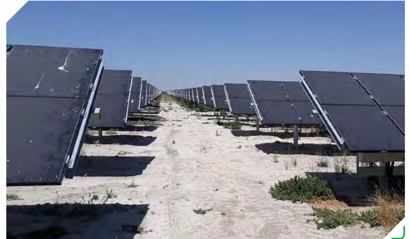
► Konya Karapınar Ges Project, Scada building, all mechanical manufacturing and engineering calculations.
